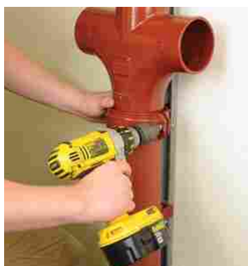
3. Push the second pipe or fitting into the coupling again ensuring that the spigot is abutted against the central register.
