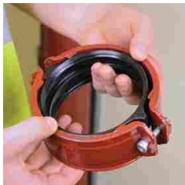
1. Slacken bolts on coupling to fullest extent to ease assembly.
